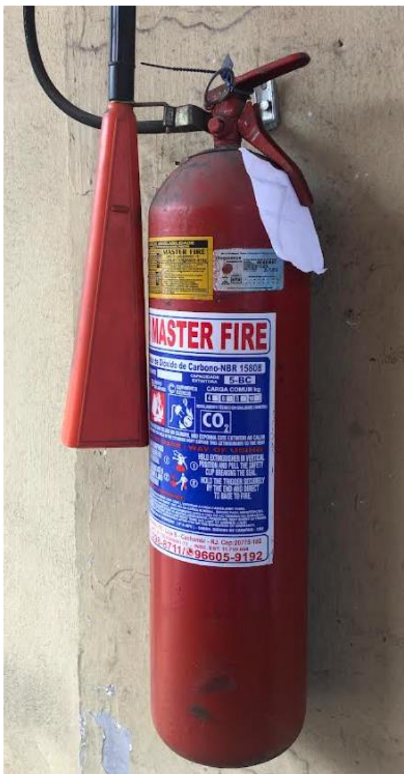
Portão Principal – Co 2
